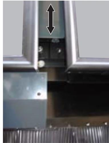
5. Insert the ball nuts into the grooves in the solar collectors in accordance with the following dimensions.
